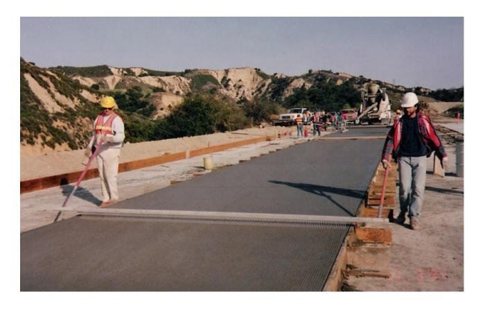
12qof ¾+spaced tines (Cal Trans Spec.) mounted on a 16qaluminum beam, comes with two 6qx 1 3/8+handles.
