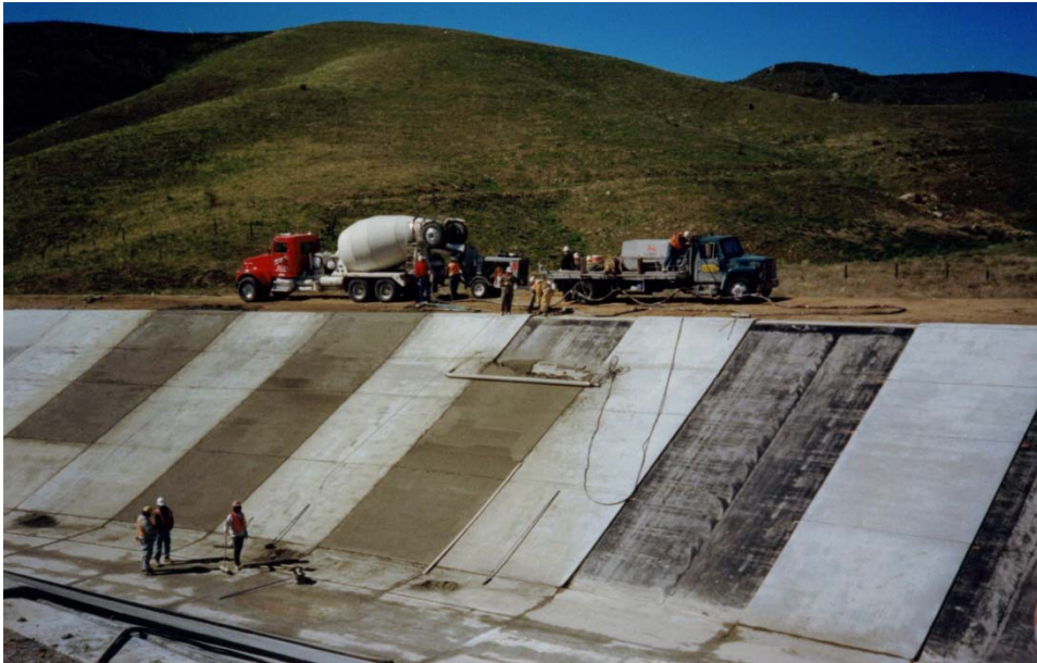
Repairing California Aqueduct with truck mounted Ditch Bank Rig
